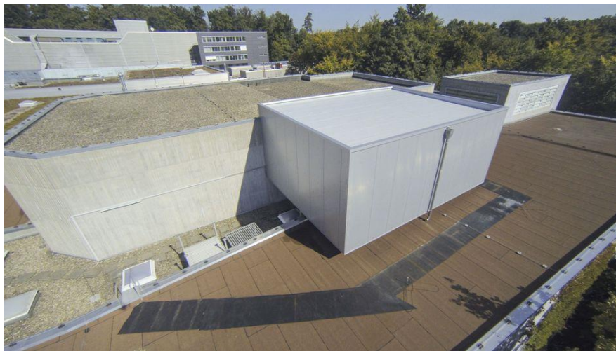
Fig. 3-7: Helmholtz resonator (gray cuboid in the foreground) attached to the wind tunnel plenum.
